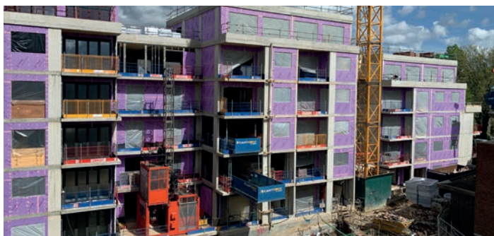
EXTERNAL PROGRESS OF THE UREN BUILDING
